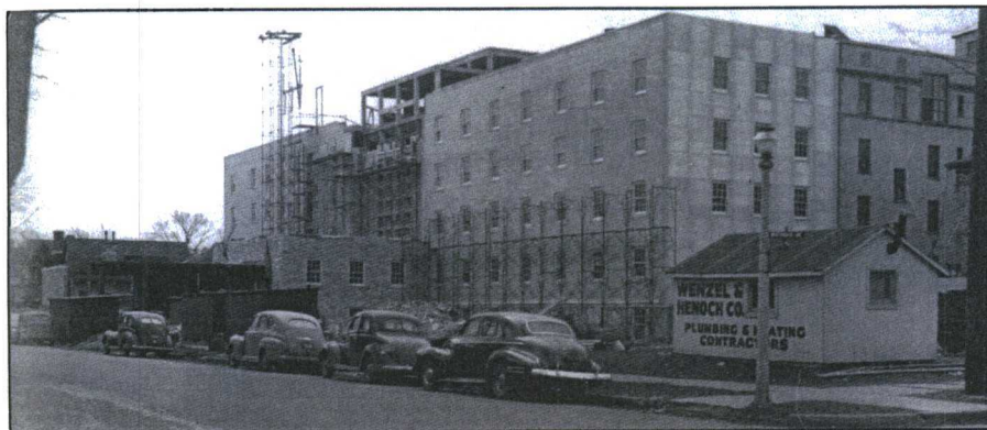
St. Luke's Hospital Addition — View from Wisconsin Avenue. Schmidt, Garden, & Erickson, Architects. Bondgard Construction Company.
